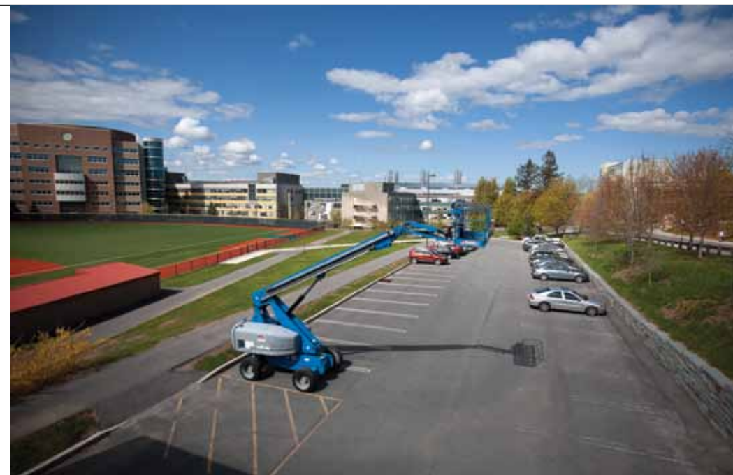
Hoy north parking lot at Hoy and Campus roads is the site for the future William H. Gates Hall, which is expected to be completed in April 2014. In this view, facing west, Hoy Field is visible at left and Rhodes and Upson halls are in the background.
